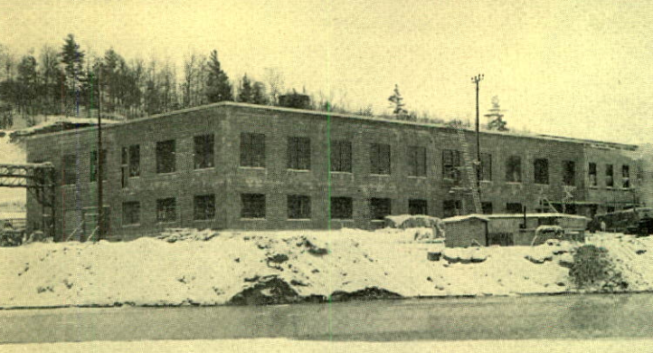
The new Finishing and Shipping Room extension at Windsor Mills
