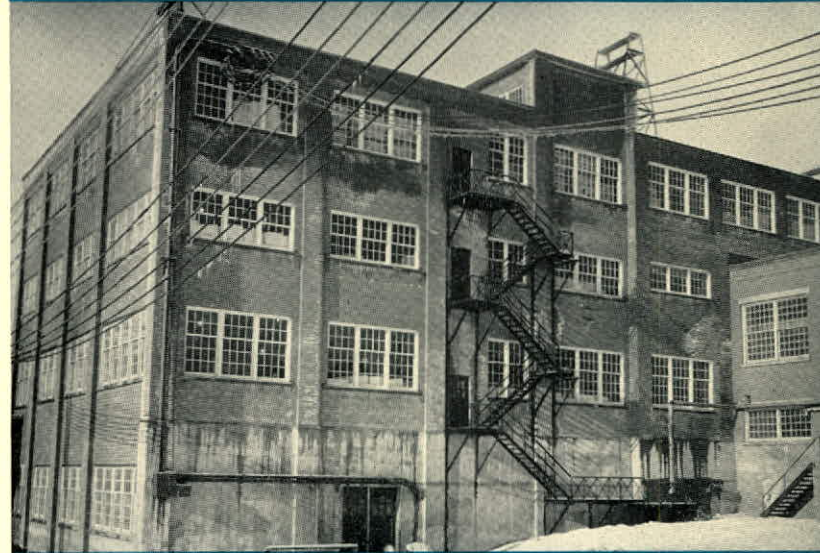
This extension to the Stock Preparation building in the Cornwall Division contains 24,000 square feet of floor space on three floors and a basement housing the necessary pulpers
