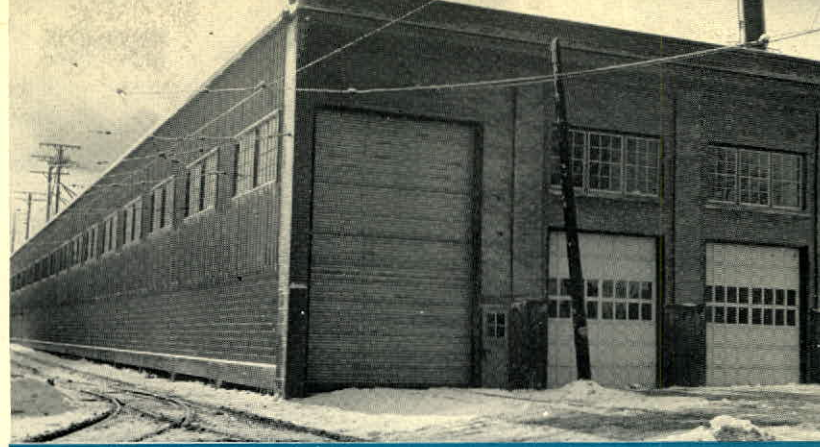
Outside view of the new Soda Pulp Shipping and Storage building. Has storage space of 14,000 square feet, and will accommodate nine boxcars and two highway transports. A series of offices are located on the mezzanine floor, including the Soda Mill Laboratory
