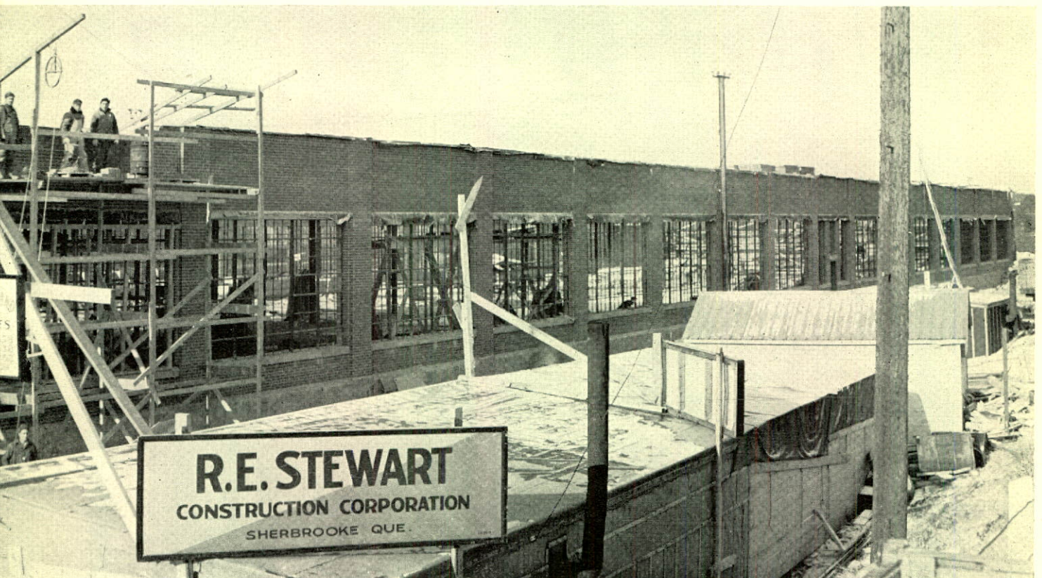
Addition to the Converted Products Division, Windsor Mills.
