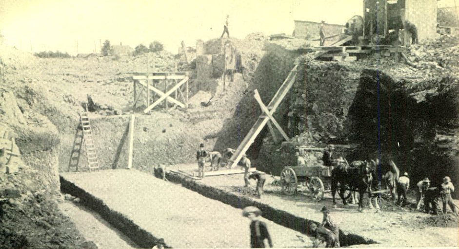
Digging the foundations for the old Lincoln Mill at Merritton.
