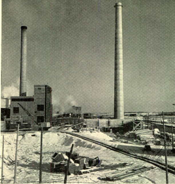
New Power Plant and Stack at Cornwall Division
