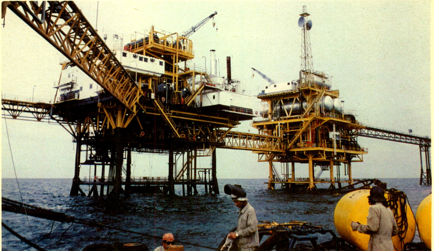
A sea-level view of the Cinta production platform in the Southeast Sumatra contract area.
