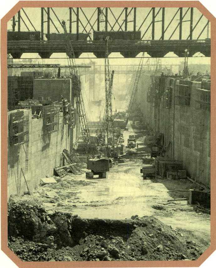
St. Lambert lock under construction, August 1957
