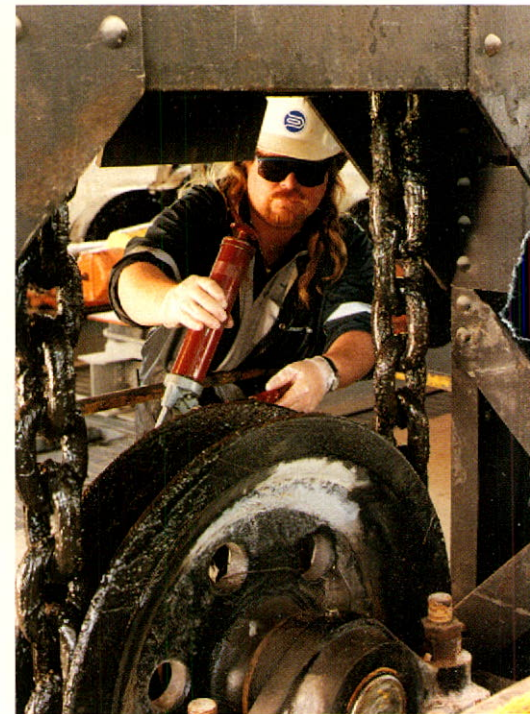
Dave Berry, Service Person, greasing the wheels that open up the locks at Lock 5, Welland Canal
