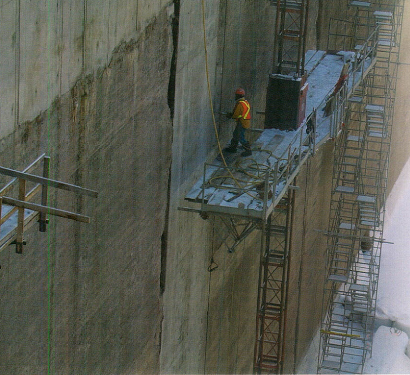
Contractor refacing lock wall during 2005 winter works
