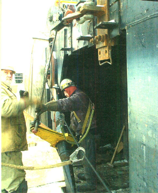
Gate rehabilitation on the Beauharnois Locks.
