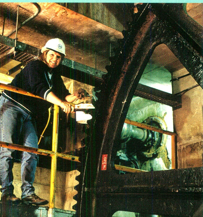
Marjorie McCullough, Service Person, painting gears that move the gates at Lock 1, Welland Canal
