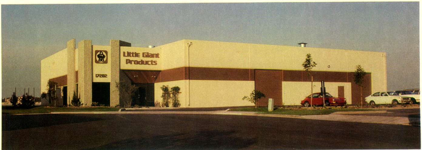
Little Giant Products’ plant in Fountain Valley, California.
