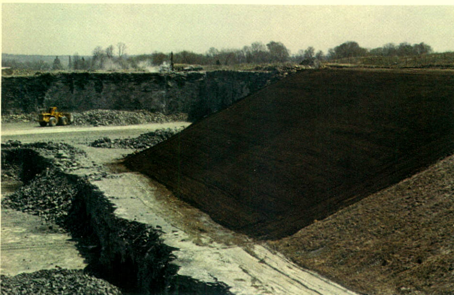
Progressive rehabilitation is taking place at the Brechin Quarry while extraction operations continue in the background.
