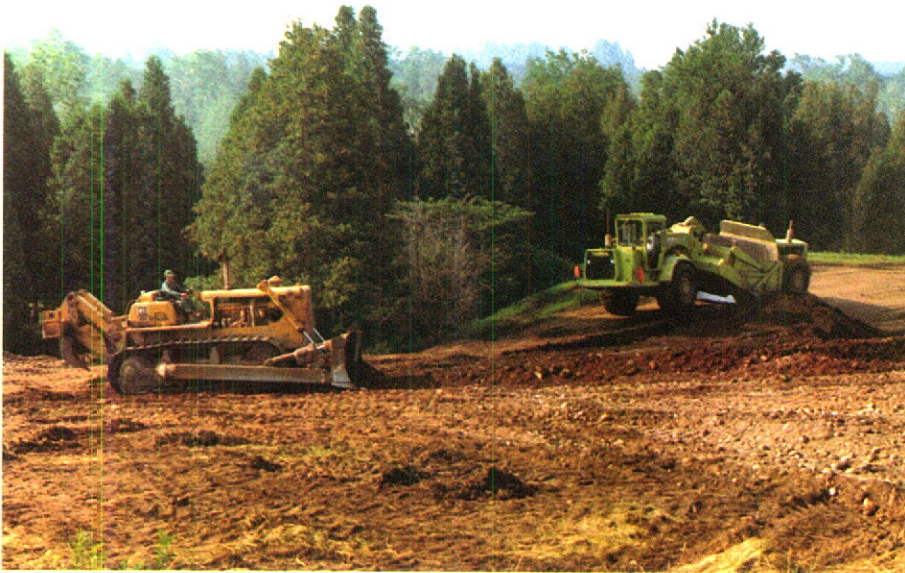
Removal of overburden to allow extraction of useable material.
