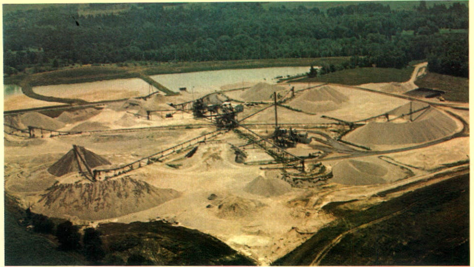
This view of the Guelph plant shows a typical layout for a sand and gravel operation.
