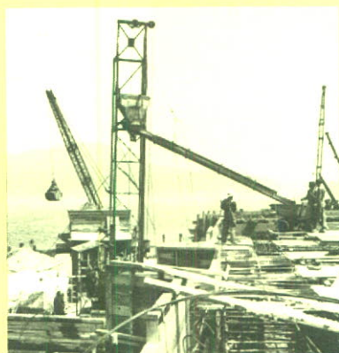
Construction of reinforced concrete dock at Westridge, July 1958.
