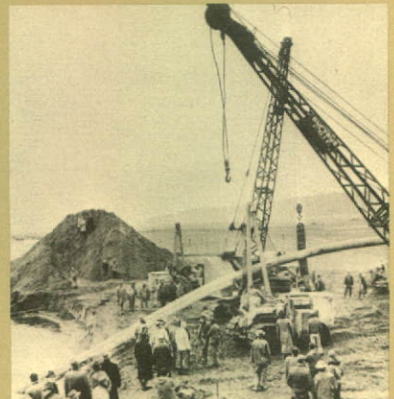
Pulling of 16 inch pipe across Swinomish Slough to Anacortes, March 1955.
