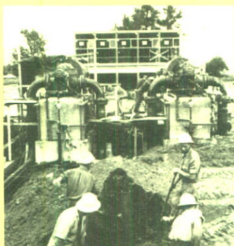
Sumas Station under construction, August 1957.
