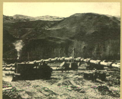
Pipe is coated and weighted for Thompson River crossing, April 1957.
