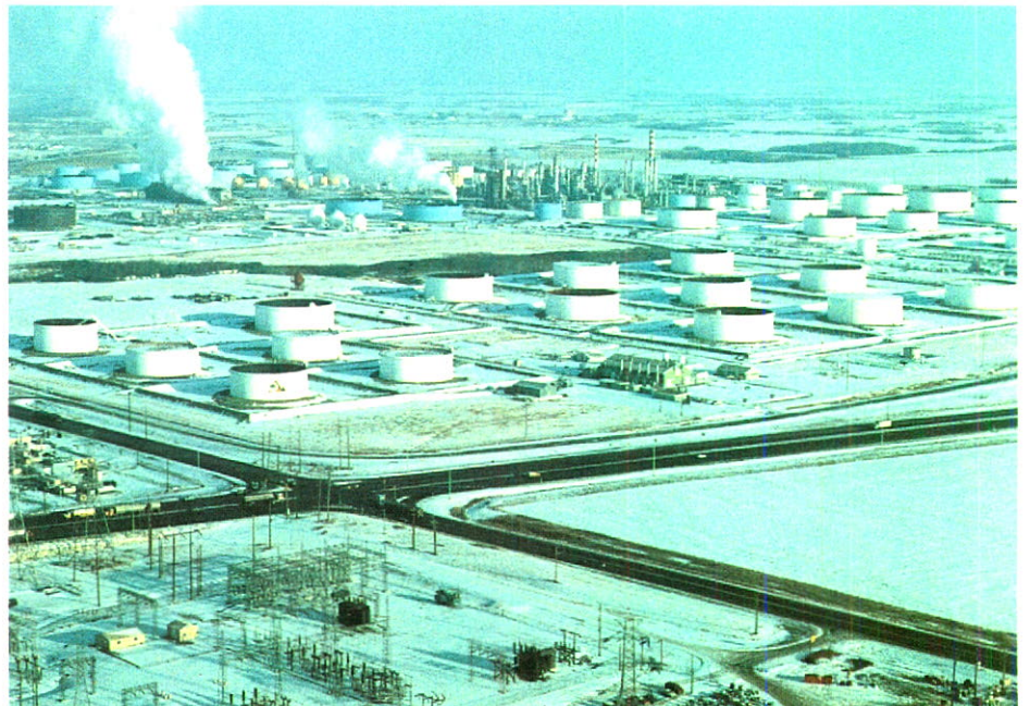
TRANS MOUNTAIN EDMONTON TERMINAL — DECEMBER, 1981
