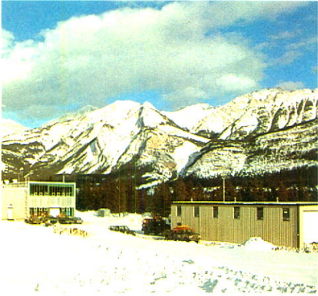
Pump Station and New Pipe Line Maintenance Garage — Jasper
