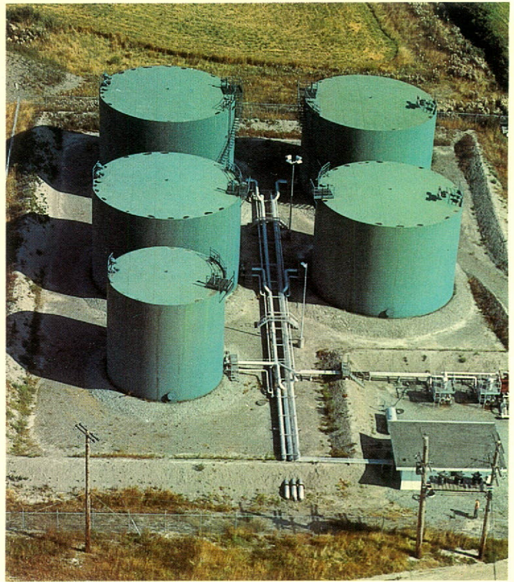
The Trans Mountain jet fuel pipe line downstream terminal is located on Sea Island adjacent to the airport.
