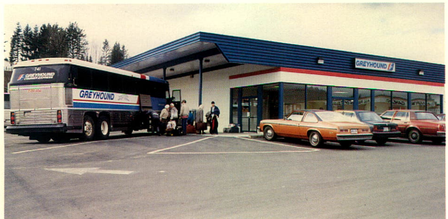
New Abbotsford, B.C. terminal was completed in 1988.
