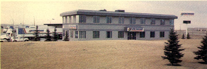
New cross-dock facility in Calgary is located near the International Airport.
