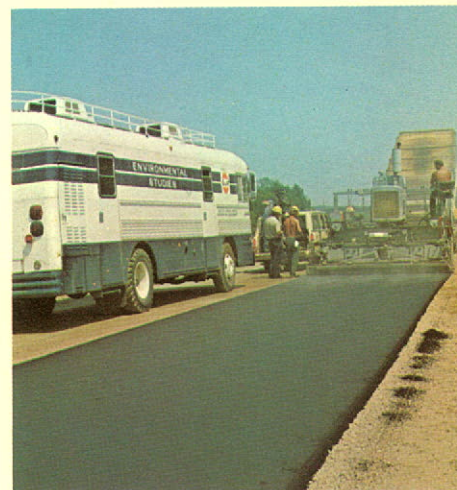
Gulf Canada's process, in which sulphur can replace up to half the asphalt binder in highway construction, is tested on an experimental road near Renfrew, Ontario.
