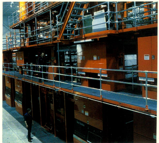
New Colorliner press being installed at the Times-Colonist, Victoria, British Columbia.
