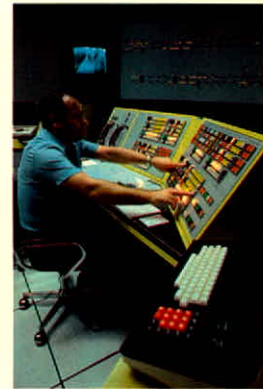
The traffic control system of the Rome subway's second line has been implemented with a PDP-11 computer by Ansaldo, one of Digital's first customers in Italy and a leader in automated systems for plants, energy and traffic control. The new subway, which tunnels through sites of the ancient Roman metropolis, involved a unique meeting of the computer age and antiquity. A young Bacchus (First Century A.D.) discovered during construction is now being restored at the Museo Nazionale di Roma.
