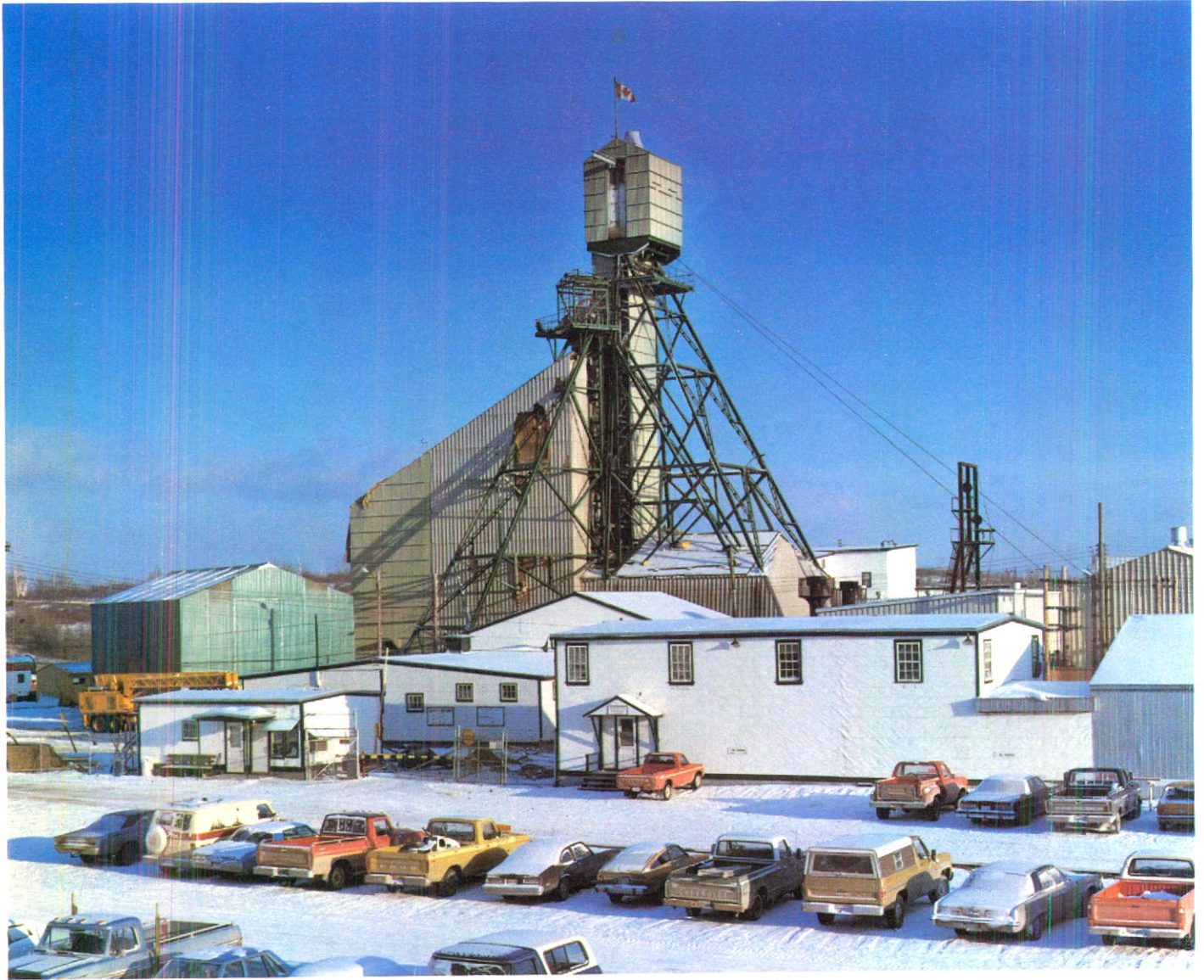
Newly modified headframe – Dickenson Mines
