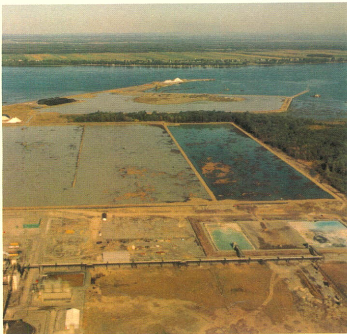
Port extension currently underway at Bécancour, Québec.
