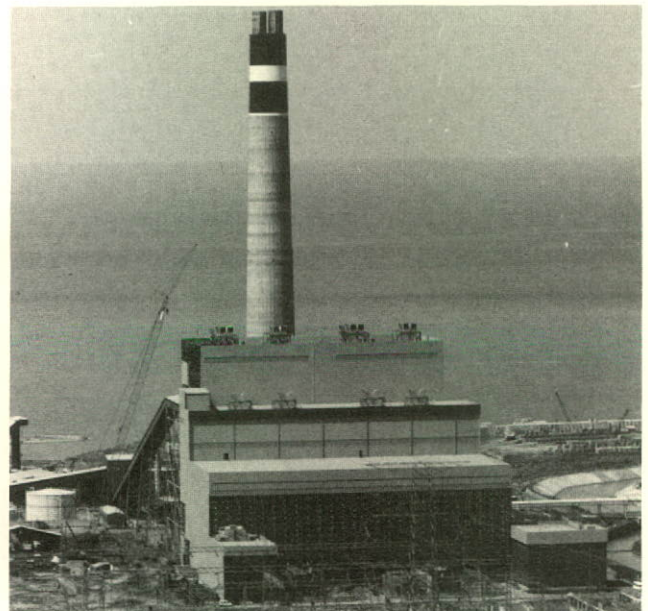
Suralaya Thermal Power Plant, Indonesia.
