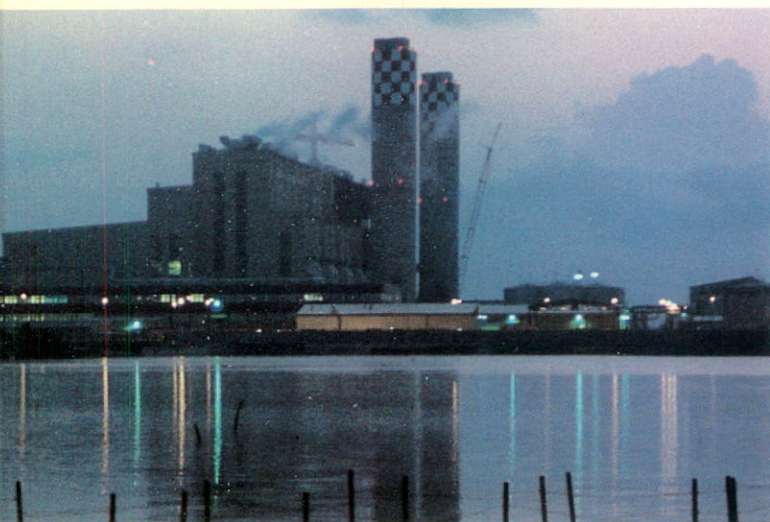
Monenco exports its advanced thermal power knowledge to Nigeria where it is designing and managing the construction of the 1320 MW Lagos Thermal Power Plant.
