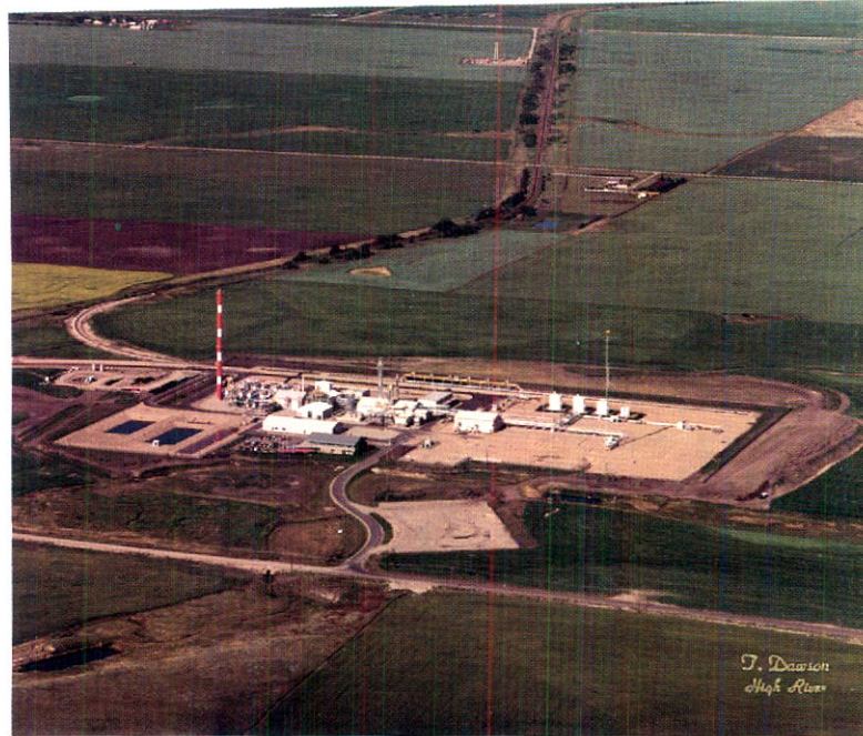
Mazeppa Gas Plant in Alberta.
