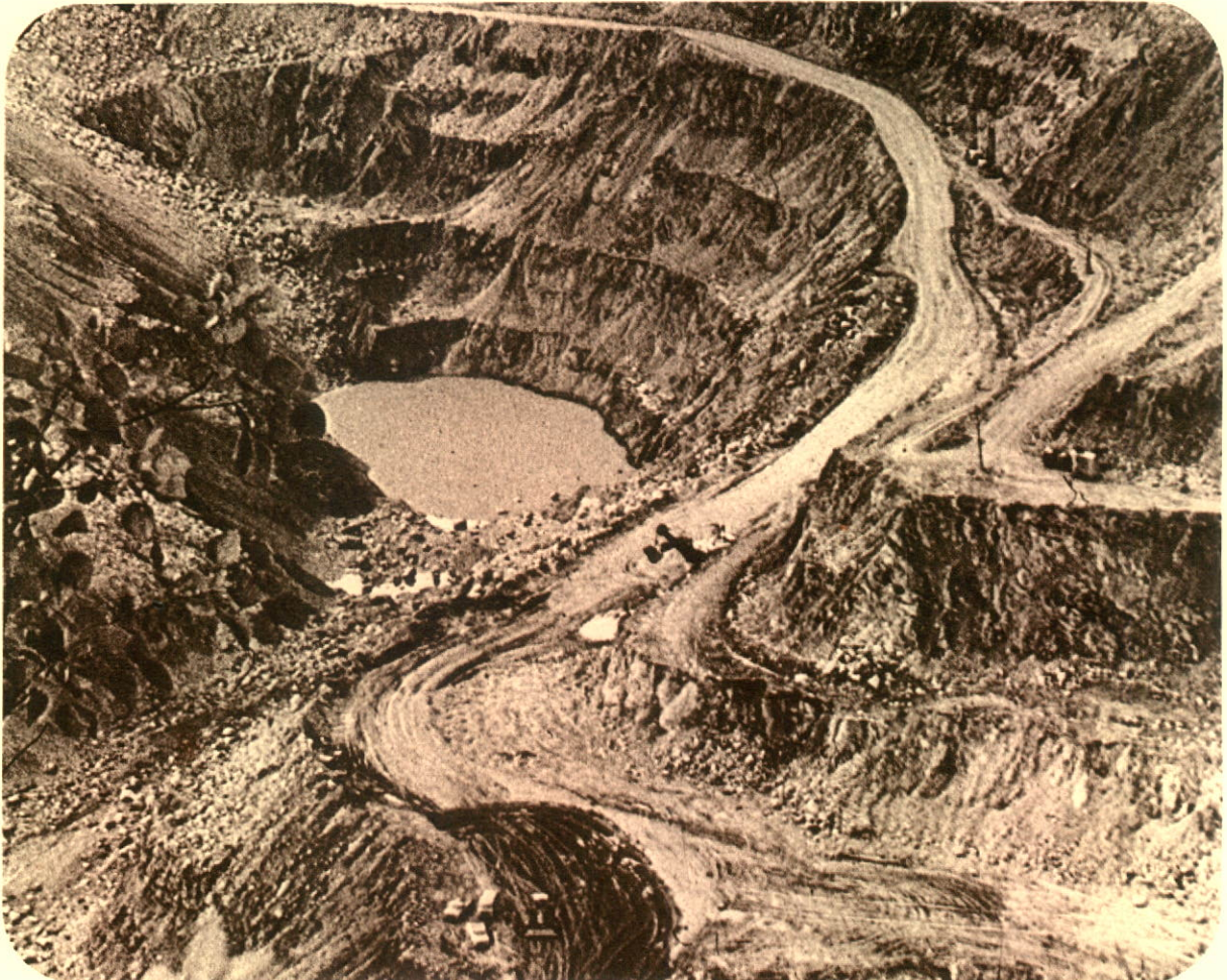
Hogarth Open Pit looking south-east
