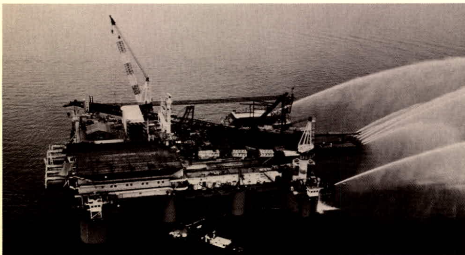
The world's most advanced sea-borne fire fighting and emergency support vessel, the MSV Tharos, entered service for the Occidental North Sea consortium early this year to provide protection for the group's offshore interests.
