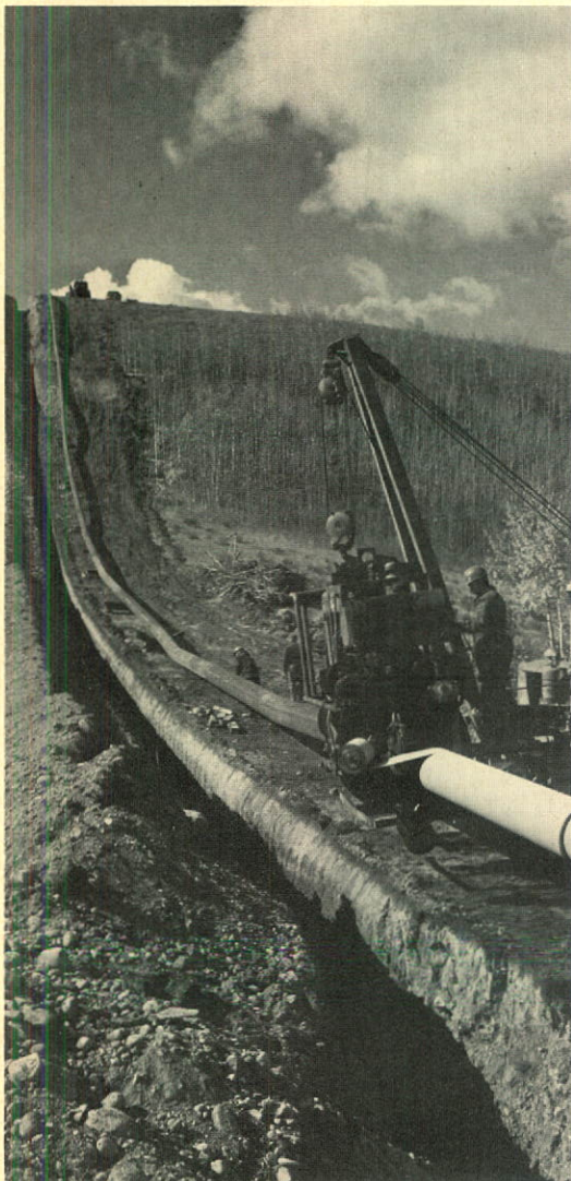
Left: Wrapping of pipe prior to installation in Canadian Western's major pipeline project for 1966 - connecting Calgary to the Jumping Pound West Field, 45 miles west of that city. Centre: Skids of explosives being pulled into Bow River west of Calgary to blast a trench bed for pipeline. Right: Plume of water shoots skyward as explosives rip a trench six feet deep for the pipeline. Bottom: Canadian Western's new service centre in Lethbridge, Alberta, puts all company facilities in that area under one roof.
