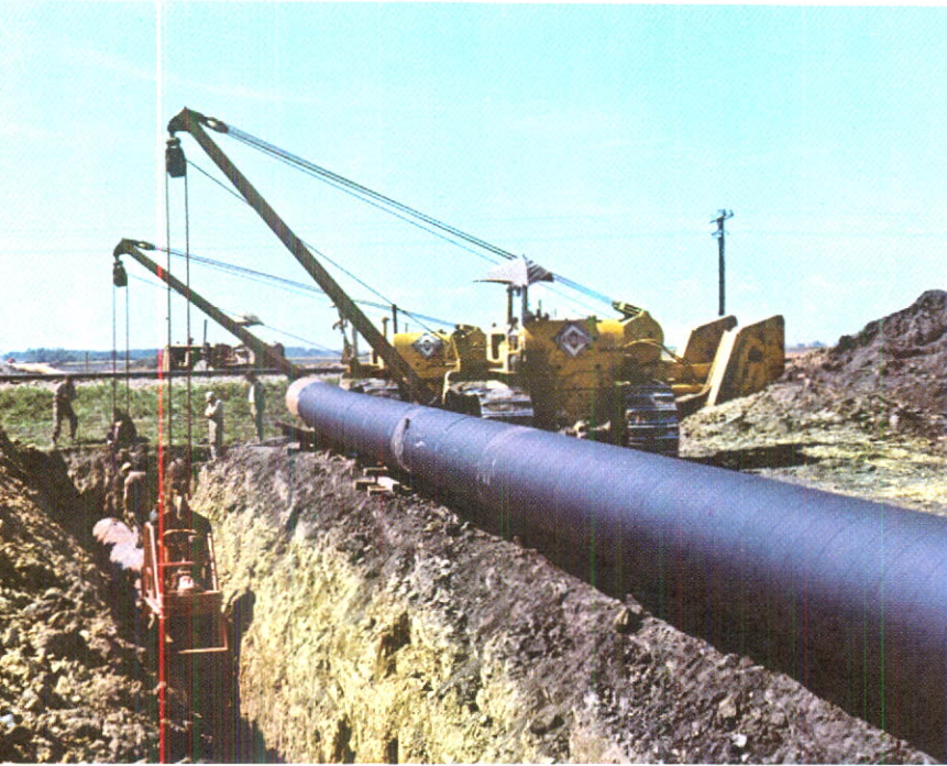
Laying 34-inch diameter pipe in Manitoba.
