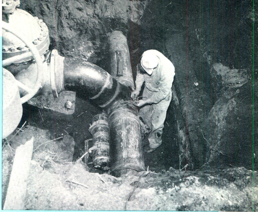
Preparing to X-ray tie-in on 16" "loop", Glenavon Station.
