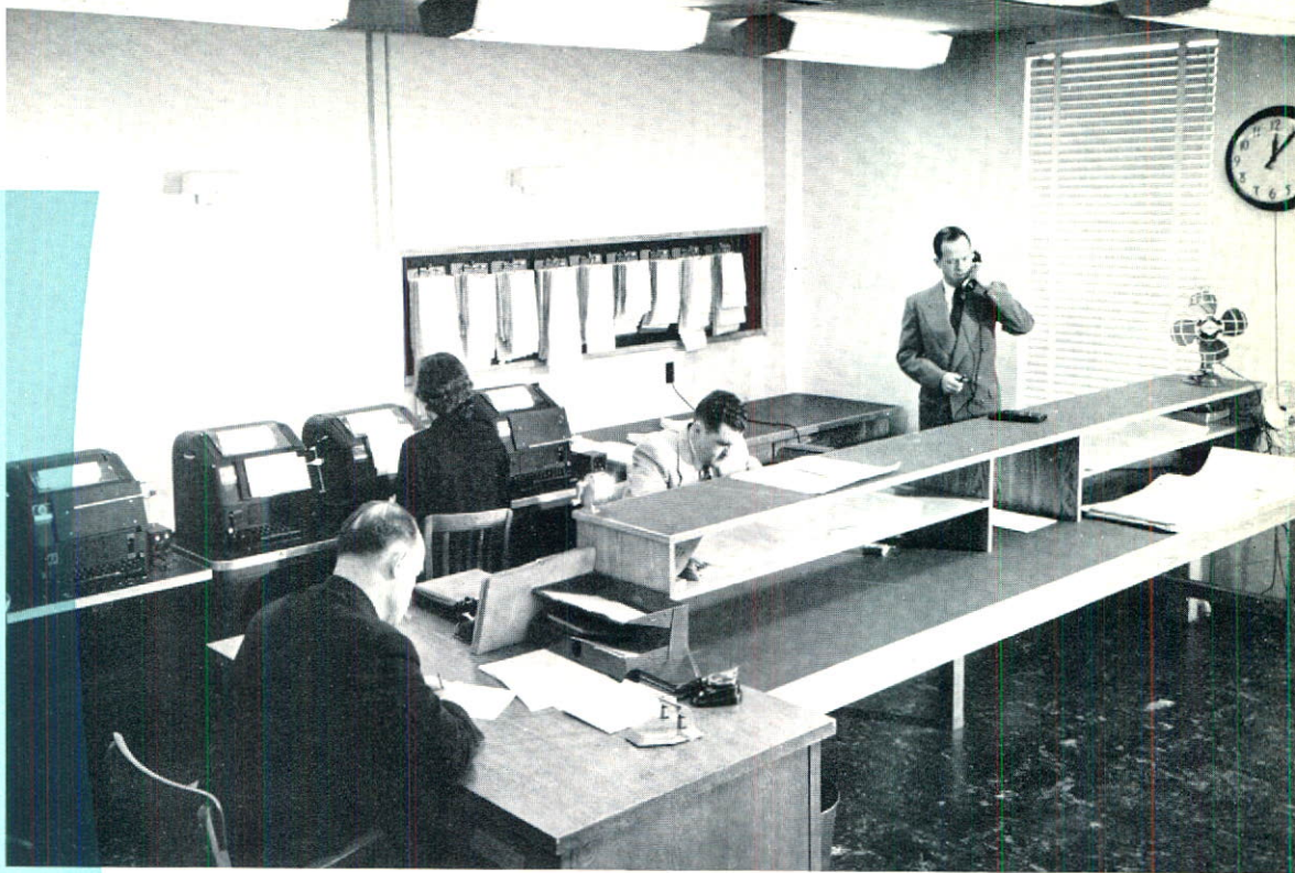
Dispatcher's office, Edmonton.
