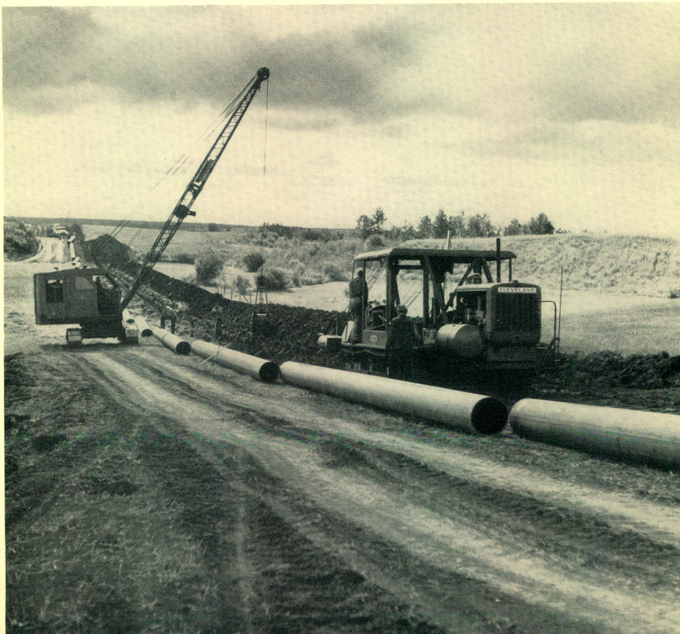
Clamshell excavators helped where ditchers encountered trouble ■
