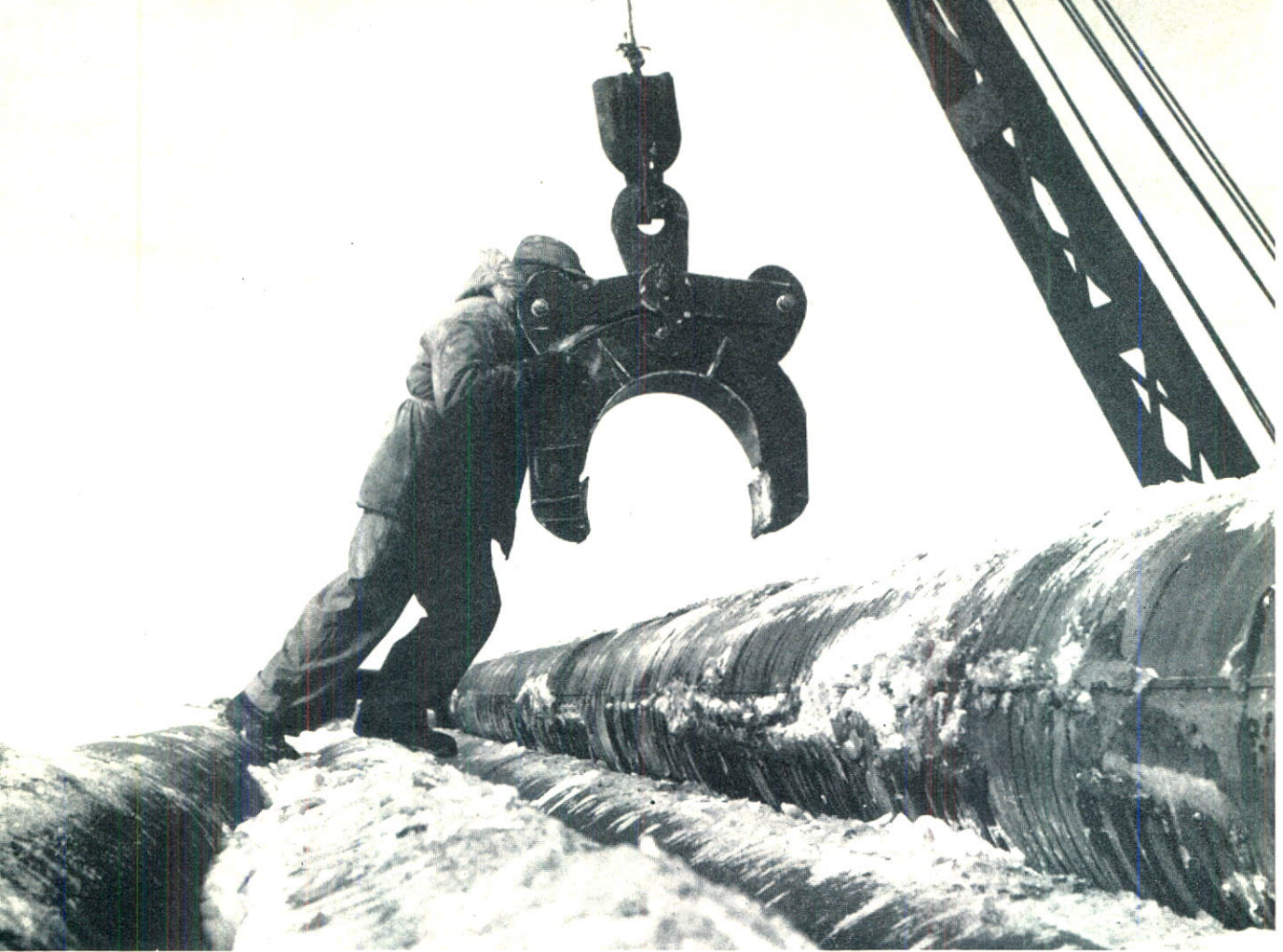
Stringing pipe started weeks before construction
