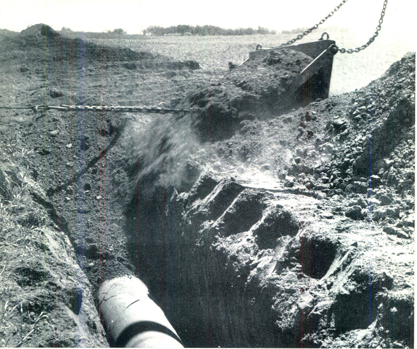
■ Backfilling did not disturb surrounding crops
