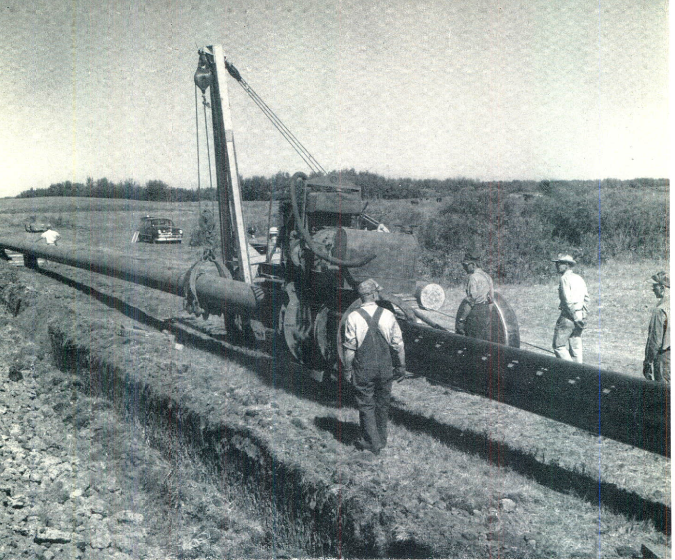
■ Self-propelled machines coated the welded pipe line
