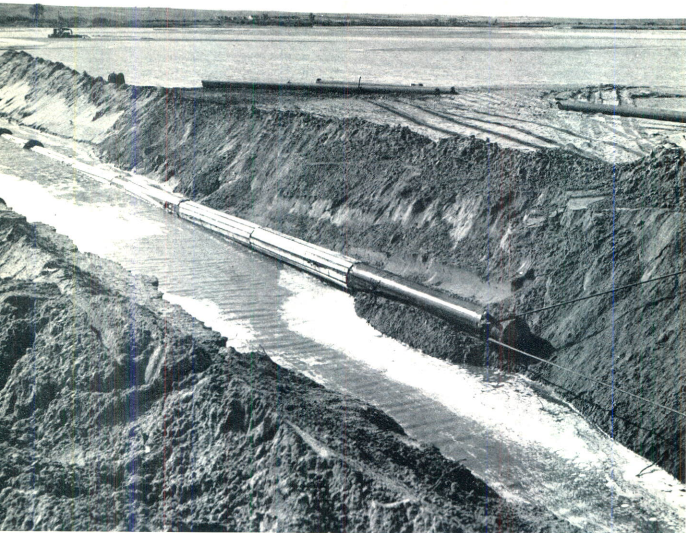
Welded pipe was floated across the Saskatchewan river
