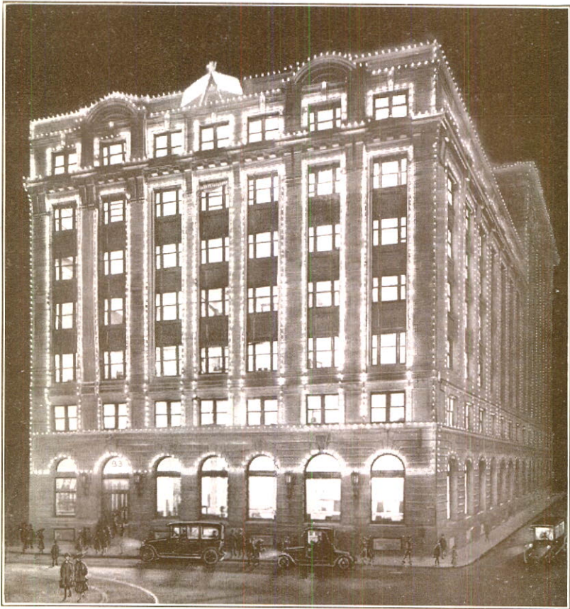
POWER BUILDING—HEAD OFFICE
