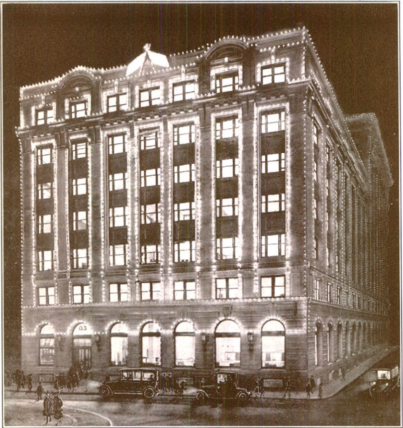
POWER BUILDING—HEAD OFFICE
