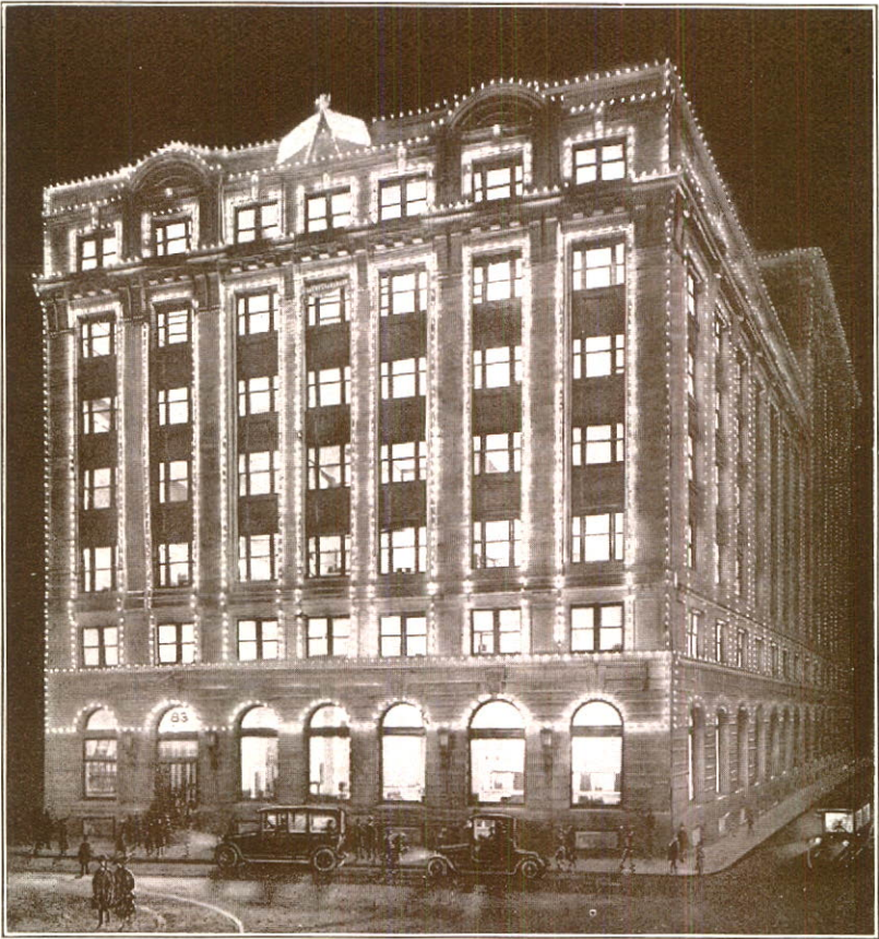
POWER BUILDING—HEAD OFFICE
