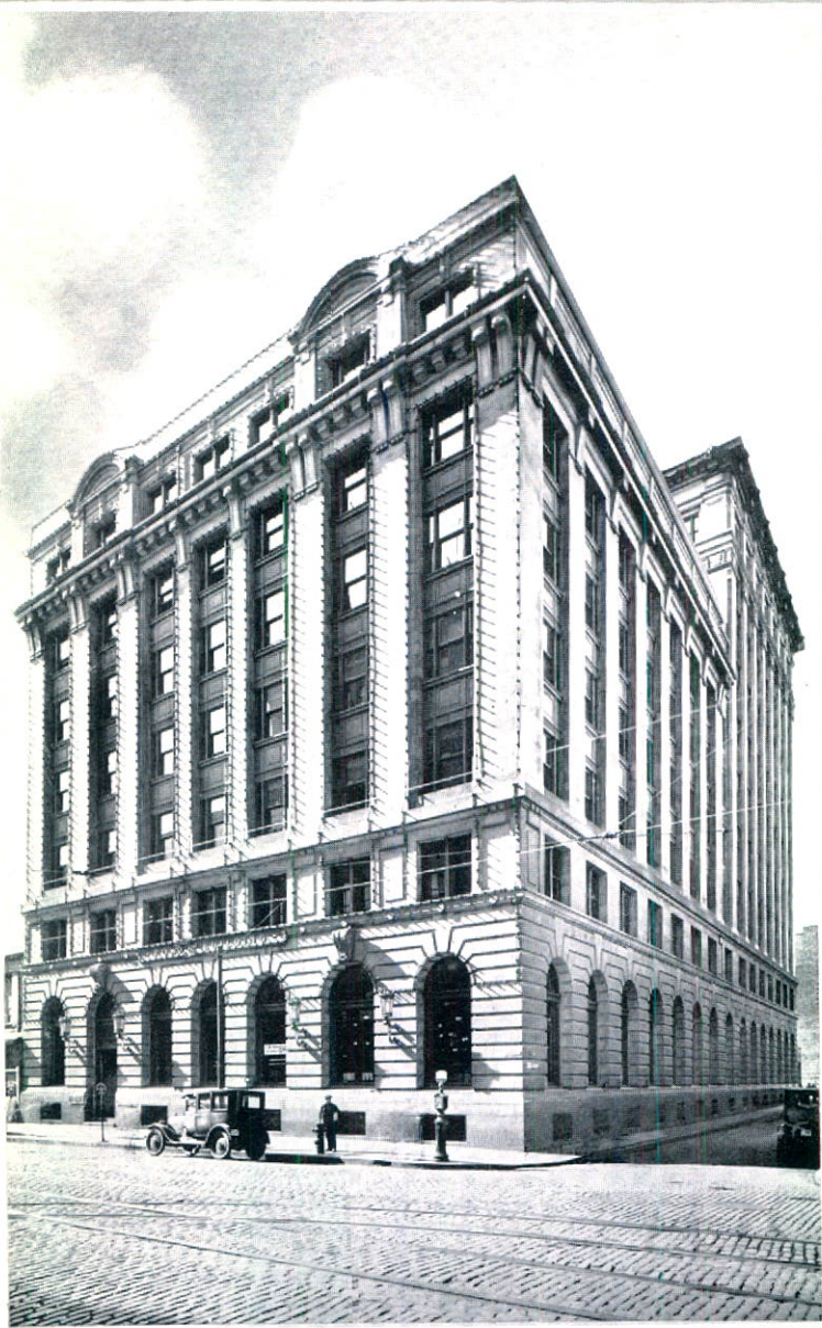
POWER BUILDING HEAD OFFICE
