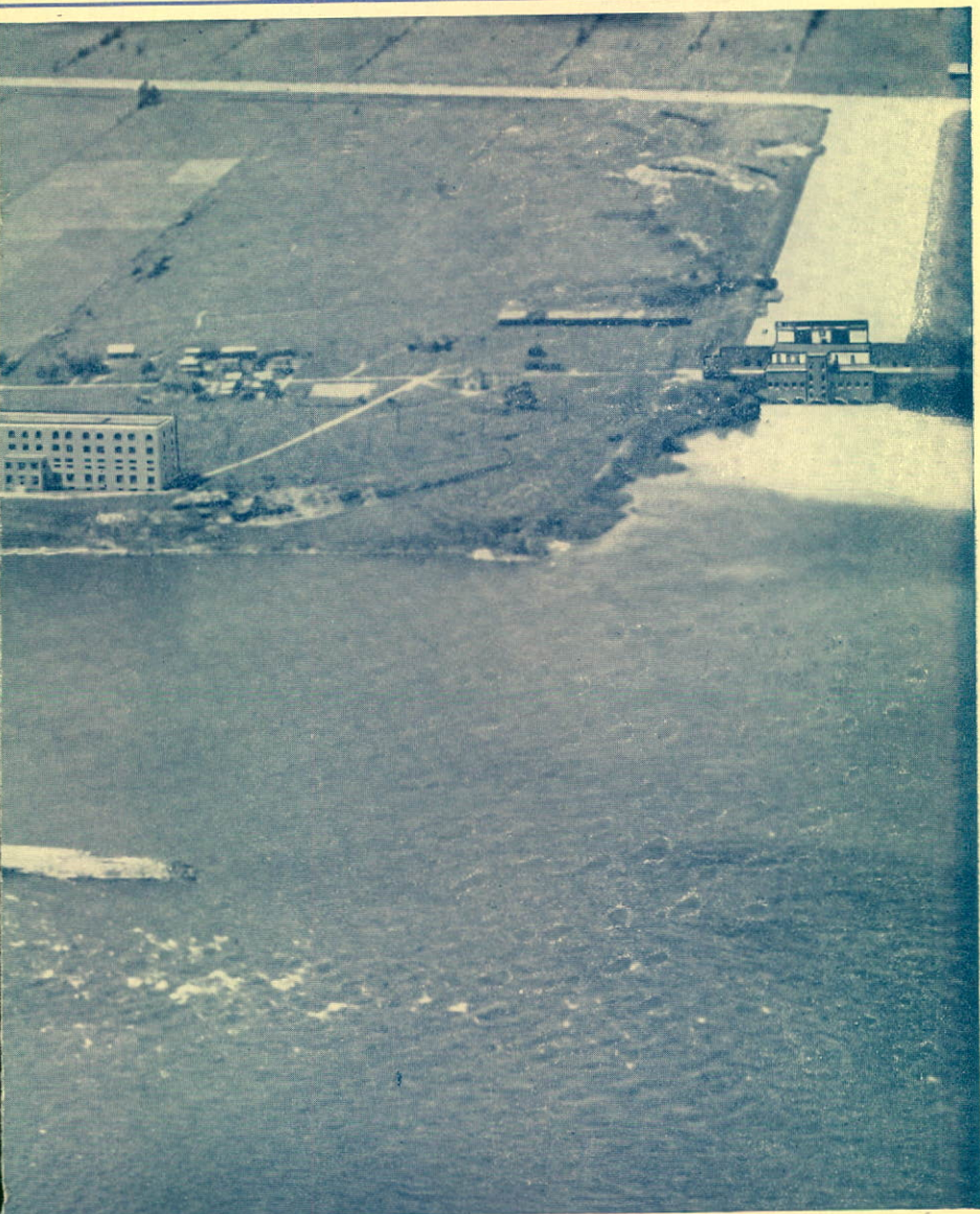
House and (right) Soulanges Power House of 16,650 H.P. installed capacity transformateurs et (à droite) usine de Soulanges (capacité installée, 16,650 c.v.)
