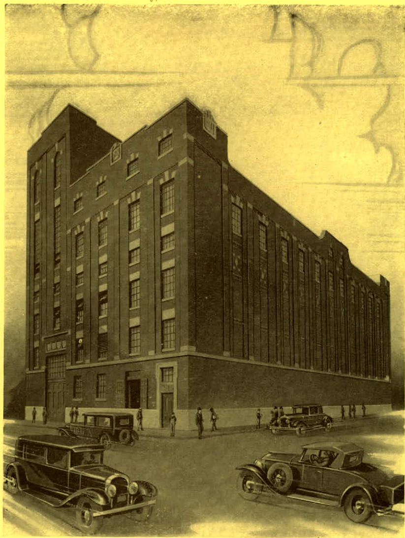
Recently enlarged Vallée Street Electric Distribution Station capacity increased to 52,500 KVA — Montreal
