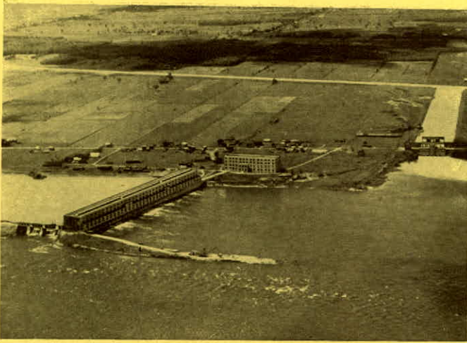
Cedars Rapids Power House of 206,400 H.P. installed capacity, Transformer House and (right) Soulanges Power House
