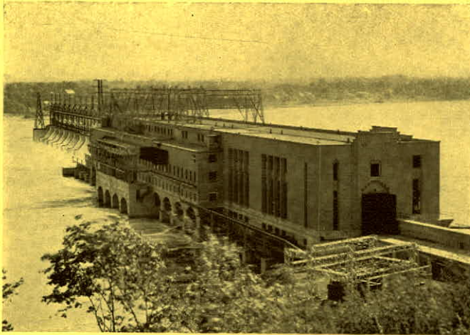
Another view of "Rivière des Prairies" Power House, with present installed capacity of 52,800 H.P.
