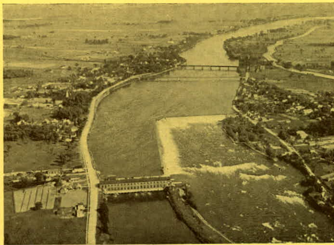
Aerial view of Chambly Power House of 22,575 H.P. installed capacity — one of the Company's earlier plants
