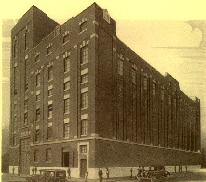
Recently enlarged Vallée Street Electric Distribution Station with capacity increased to 52,500 KVA — Montreal
