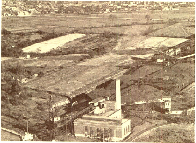
Aerial view of By-Product Coke and Gas Plant which covers an area of 120 arpents and has an annual capacity of: 9,000,000,000 cubic feet of gas; 450,000 tons of coke; 10,000,000 pounds of ammonium sulphate; 730,000 pounds of sulphur; 3,500,000 gallons of tar and 1,890,000 gallons of benzol — Ville La Salle
