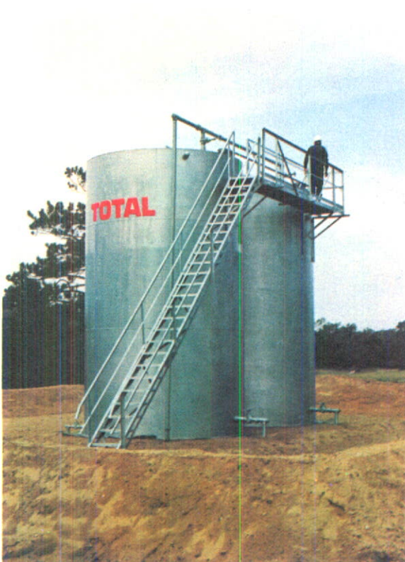
An oil storage tank on the site of the Malstrom-Williams well in Mason County, Michigan.
