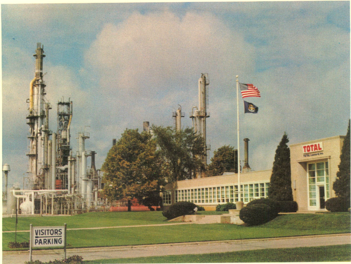
A portion of the Company's refinery at Alma, Michigan, showing the recently constructed 10,000 BPD Platformer in the foreground.
