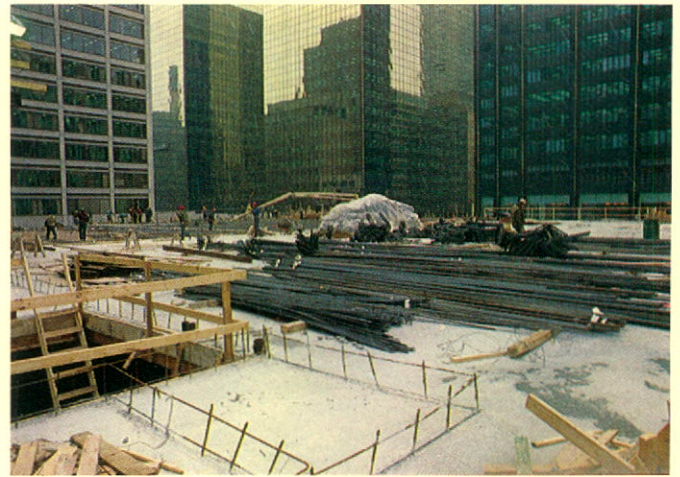
The construction site of the new trading pavilion.
