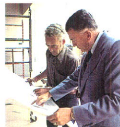
Fred Anderson reviews plans for TD's first branch in Watrous with Merle Oberg, Foreman of Bird Construction Co. Ltd.
