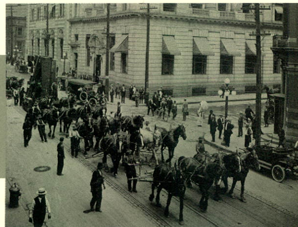
In 1914, the largest steel vault in Canada arrived at the Dominion Bank's head office at King and Yonge, Toronto.
