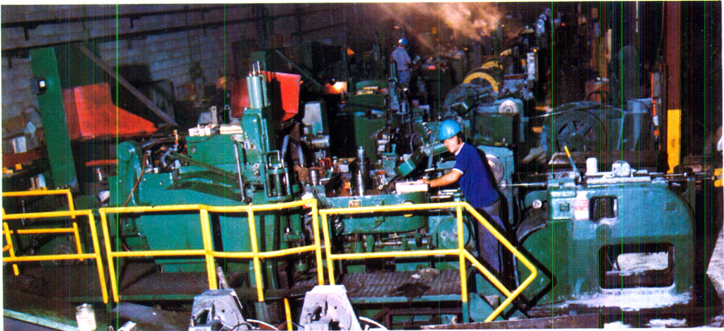
▲ High speed boltmakers in operation.
