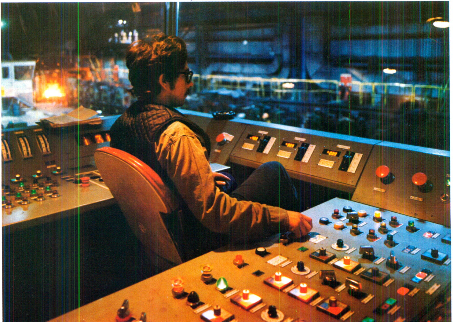
▲ It's called "the pulpit", and it's the nerve center which electronically controls each of the two strands being rolled simultaneously in the rolling mill.
