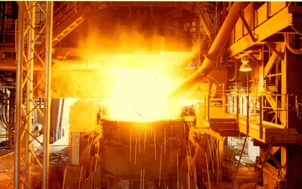
Atlantic Steel's new eccentric bottom tapping furnace, at Cartersville features automated alloy charging.
