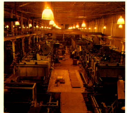
Heat treating furnaces at the Infasco Marieville plant.
