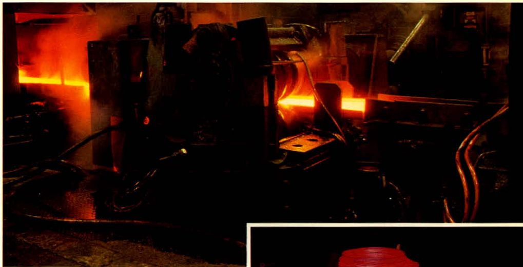
Special Bar Quality (SBQ) billet enters the descaling stands after leaving the reheat furnace.
