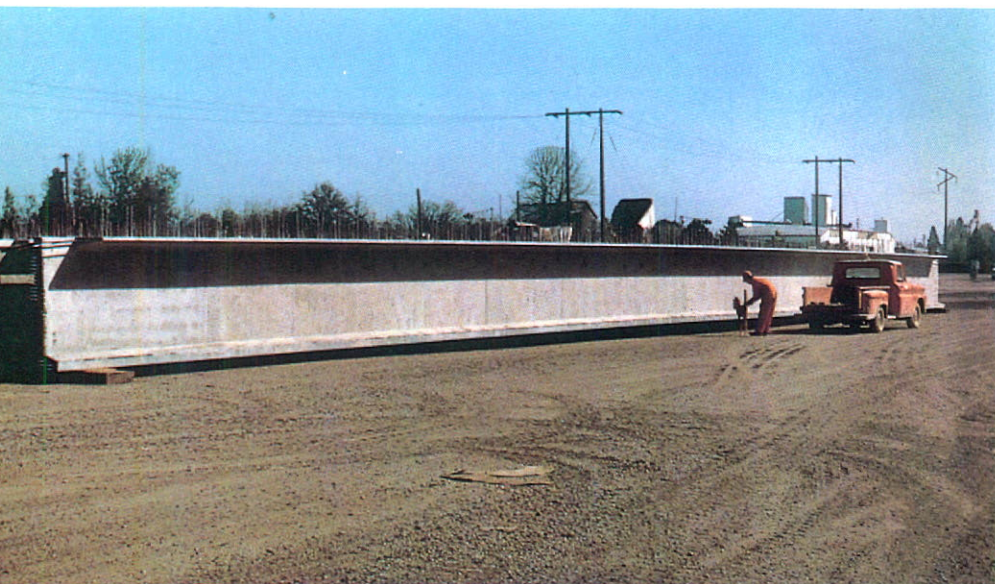
◀ A prestressed concrete bridge girder, reinforced by FLO-TECH ® , ready for placement in the Quincy Bridge in Illinois.
