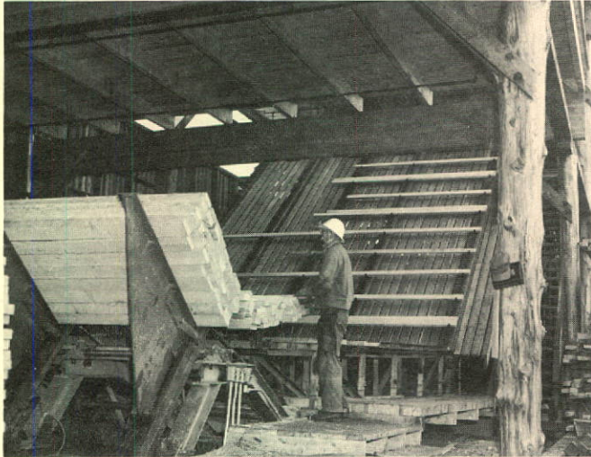
Another installation at the sawmills which has reduced labor and increased efficiency is the Setzer sorter-stacker. Random length lumber begins climb to sorter shown below.
