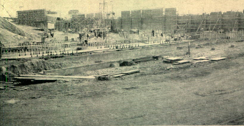
No. 9 Machine Building takes shape. New Greenwood Mill in foreground.
