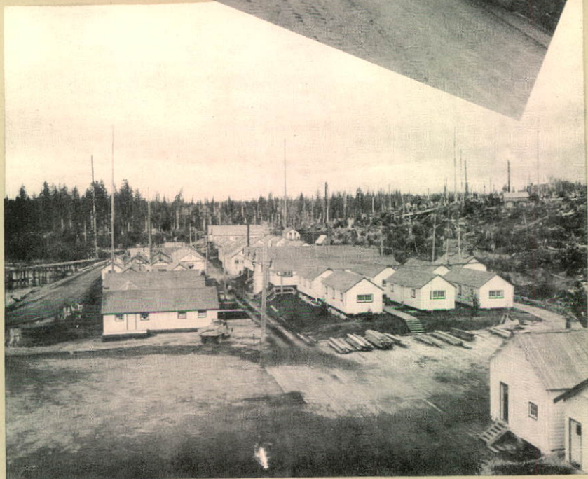
View of single men's quarters at Juskatla accommodating 250 men. There are also dwellings for 30 families at the camp. Central heating, air conditioning, hot and cold water and electric light are features of the buildings.
