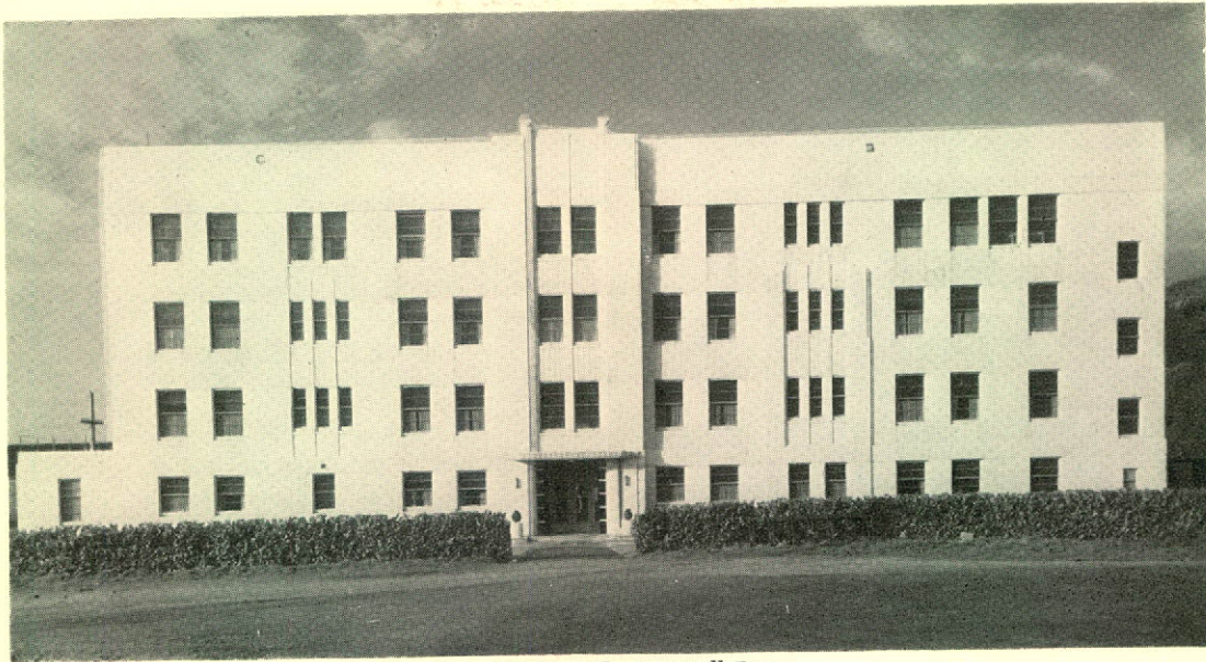
Employees' Hospital at Powell River.
