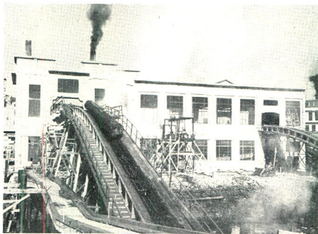
Hydraulic Barker Building during Construction.
