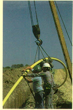
Laying pipeline in the Wood River area of southern Alberta.
